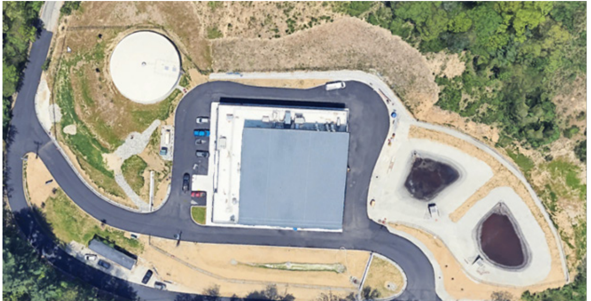
Newly Constructed Water Treatment Plant located at 18 Kimball Drive, Hooksett, NH
